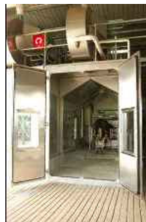
The new methane chambers at Ellinbank
